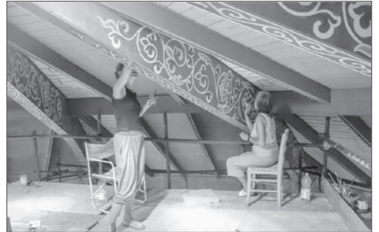
Painting the Gonpa ceiling.
