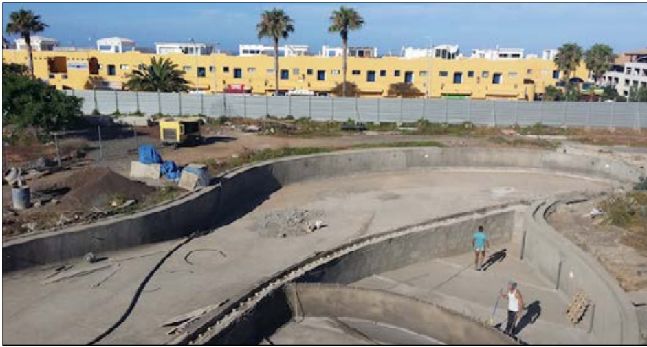
Work on the Dzamling Gar swimming pool is nearly finished with the inauguration planned for New Year's Eve.
