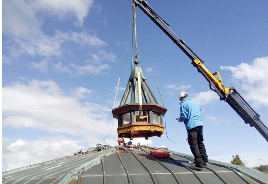
Removing the lantern from the roof.
