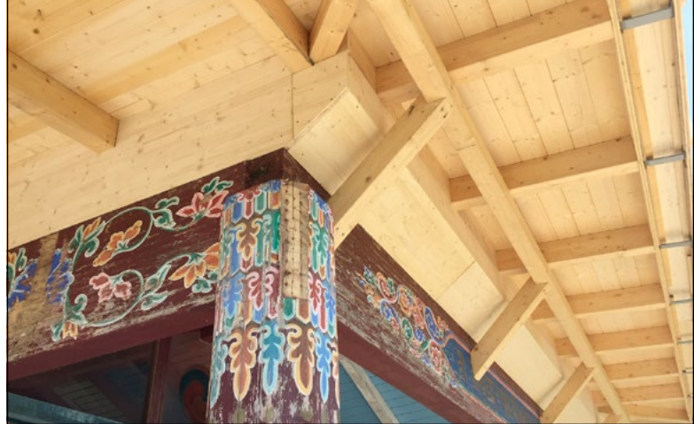
The base of the new roof extension.
