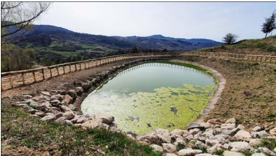
Developing water maintenance below the Yellow House.
