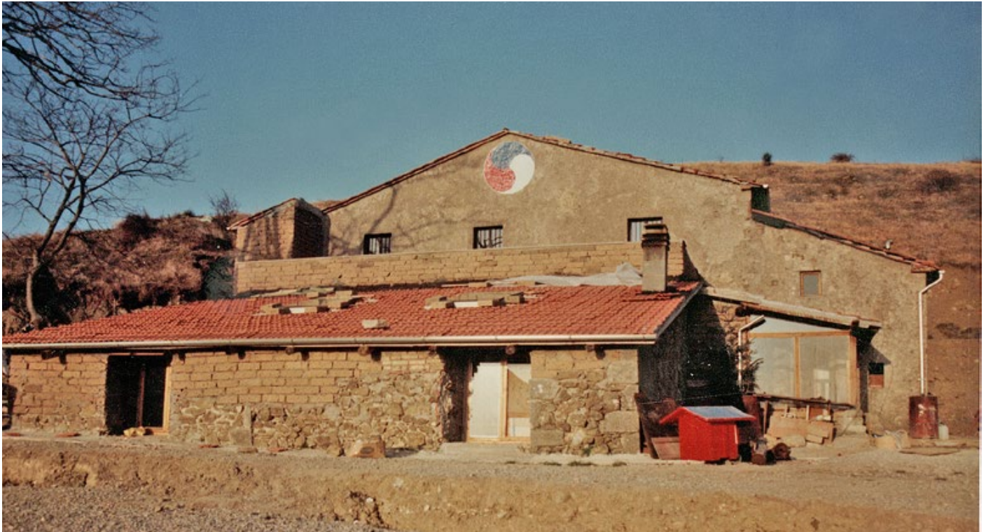
View of the ruined building that would become the Yellow House. Those of us working at Merigar at the time lived in the house while there was no roof on a major part of the building. Photo John Shane.
