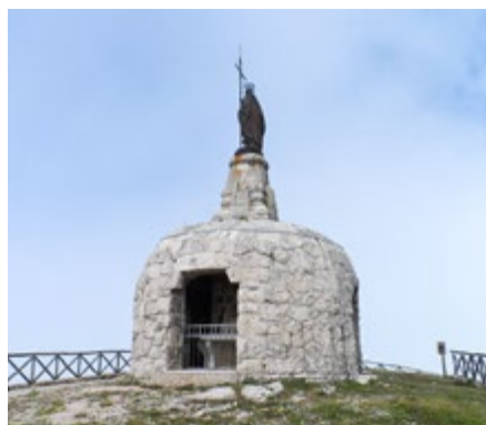
Close up of the cupola on Monte il Redentore, showing the doorway into it
